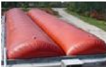
DIGESTER STORAGE TANK
